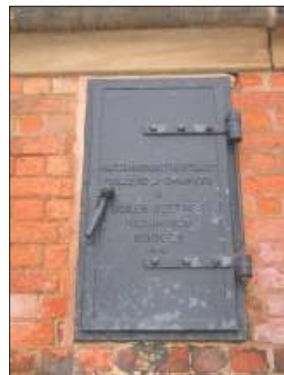
Hatch within northeastern elevation of Heritage Brewery
