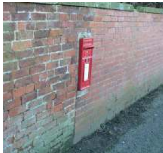
Attractive post box recessed into wall
