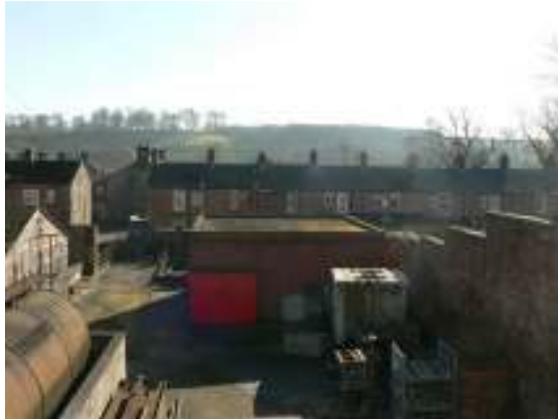
Attractive views towards the surrounding hills are visible over the workers' houses.
