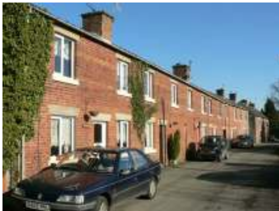
Attractive terraces properties with unsympathetic uPVC windows
