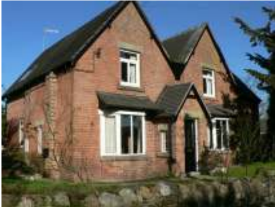
Inappropriate uPVC windows on historic properties
