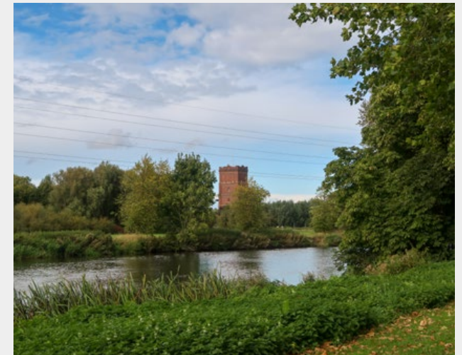
View of the Grade II Listed Water Tower, looking north-east across the River Trent
