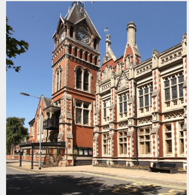
View of the Town Hall, Grade II Listed
