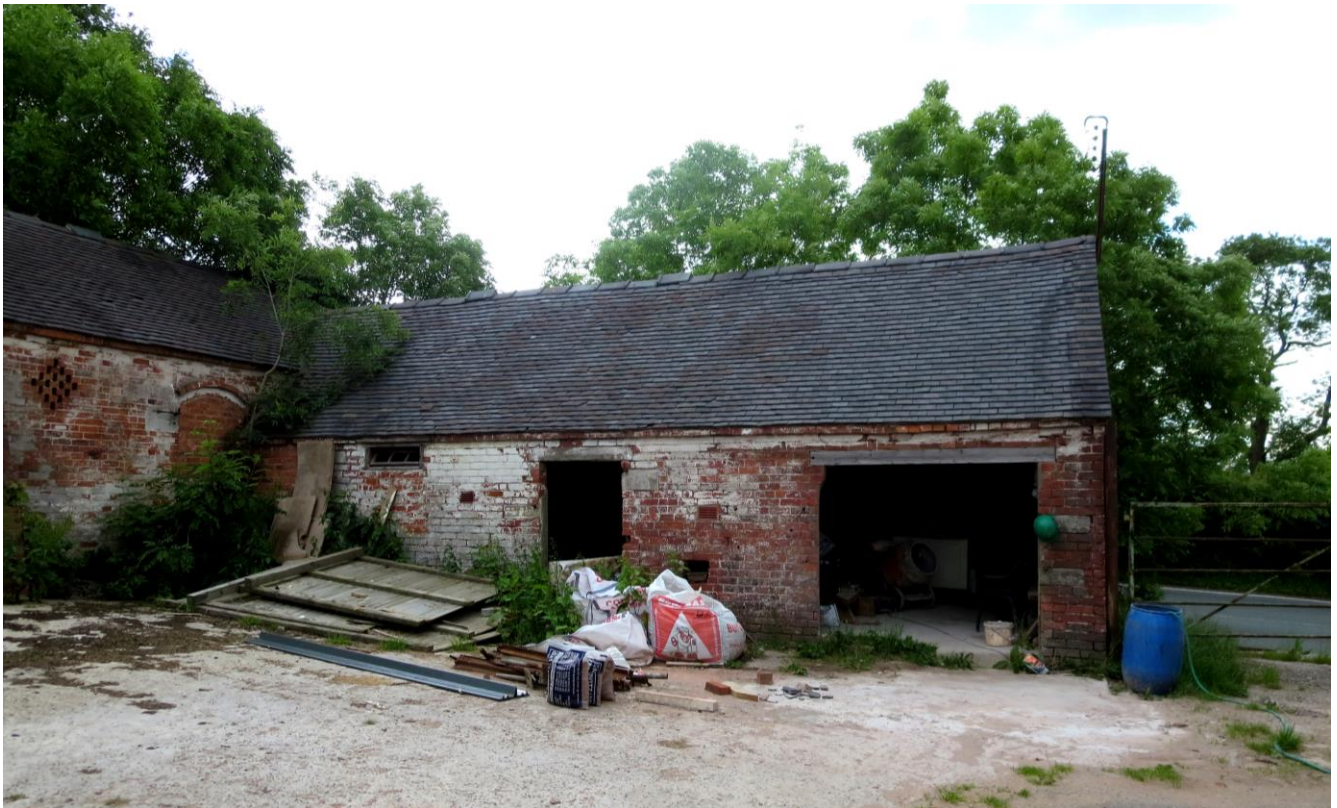
Figure 2.3 Proposed Building to be Converted (Unit 1)
