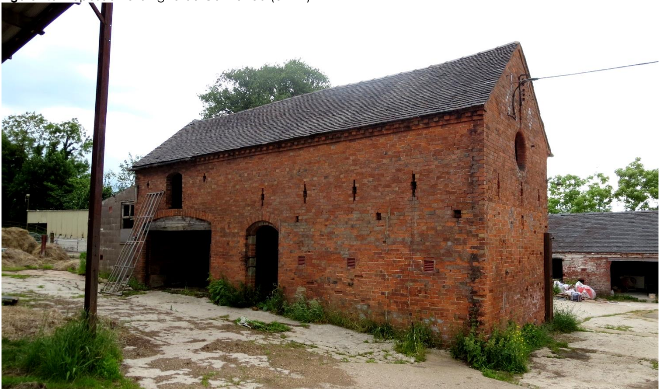
Figure 1.4 Proposed Building to be Converted (Unit 2)
