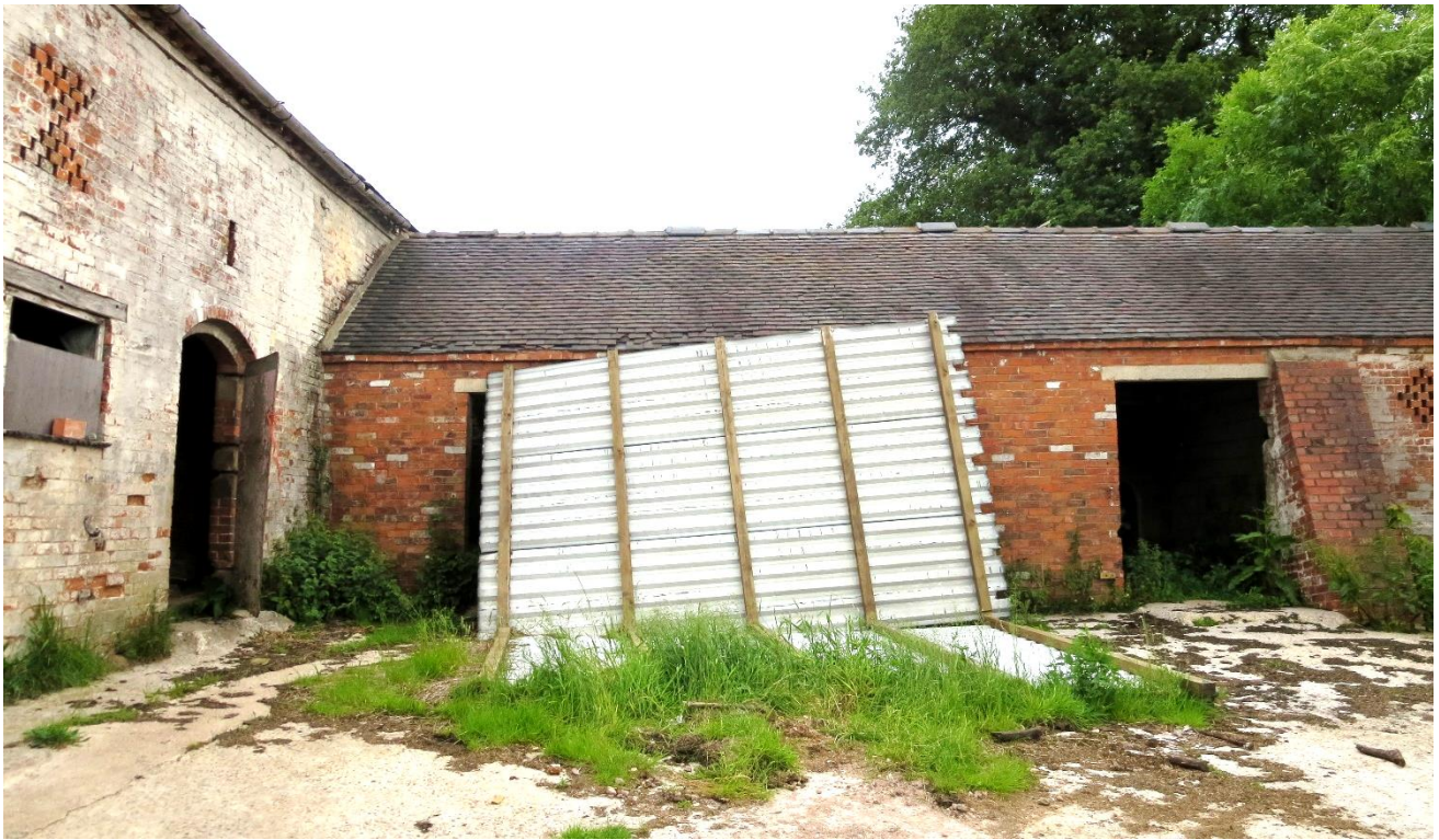
Figure 1.1 Proposed Building to be Converted (Unit 1)
