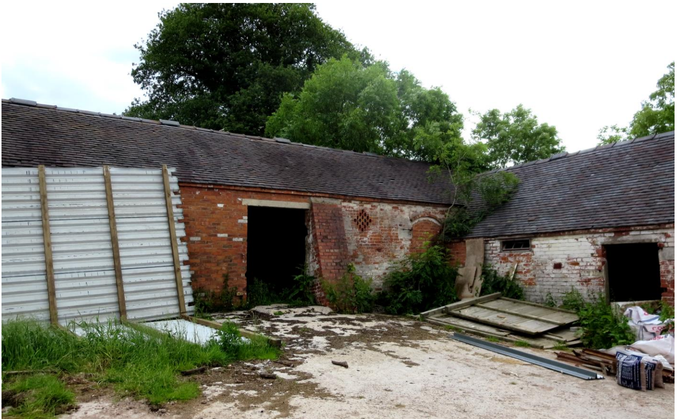
Figure 2.2 Proposed Building to be Converted (Unit 1)
