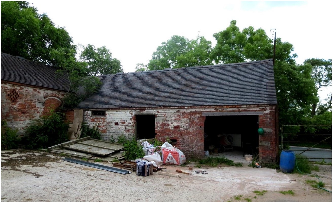
Figure 1.3 Proposed Building to be Converted (Unit 1)
