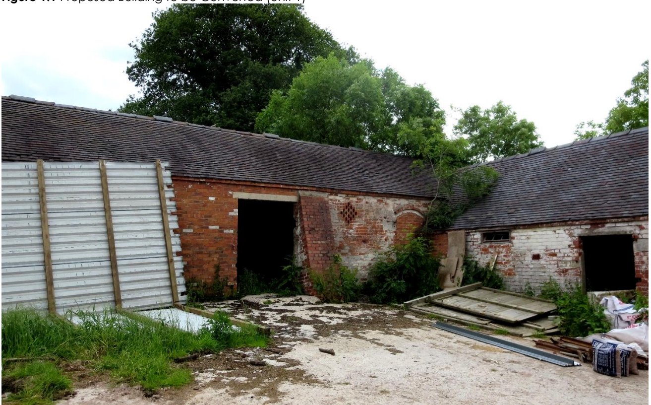
Figure 1.2 Proposed Building to be Converted (Unit 1)
