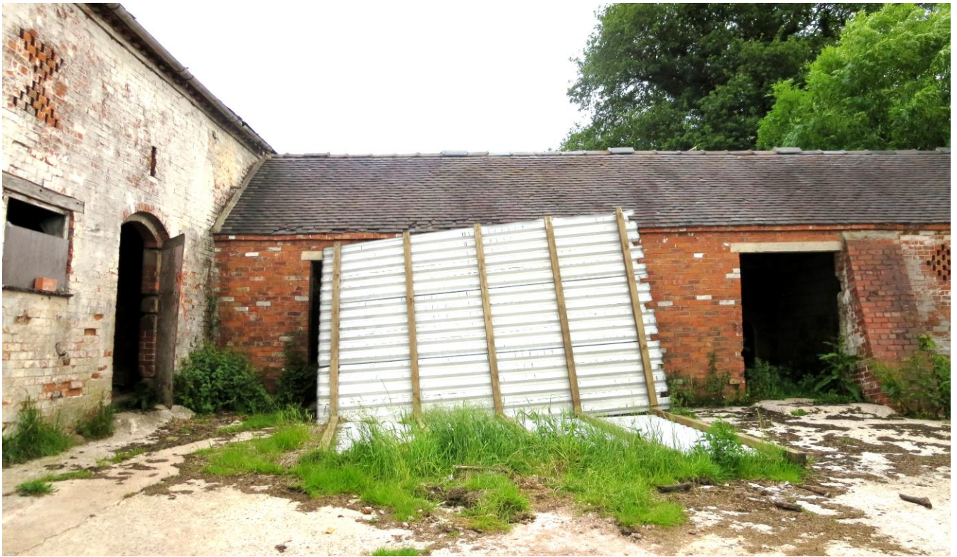
Figure 2.1 Proposed Building to be Converted (Unit 1)
