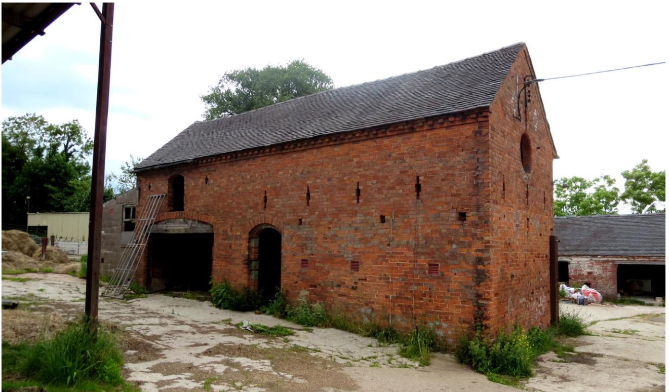
Figure 2.4 Proposed Building to be Converted (Unit 2)
