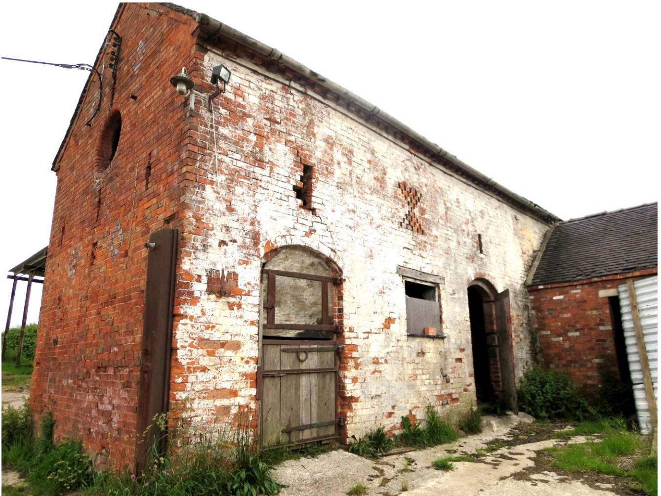
Figure 2.5 Proposed Building to be Converted (Unit 2)
