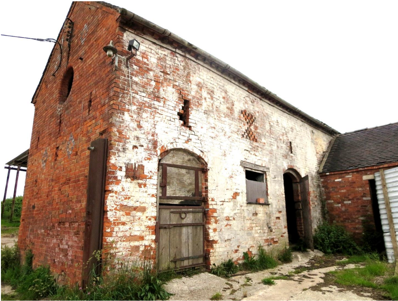
Figure 1.5 Proposed Building to be Converted (Unit 2)
