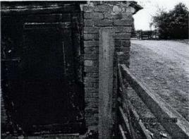
5.2.2 The right hand elevation has been reconstructed in reclaimed brickwork in recent years.
