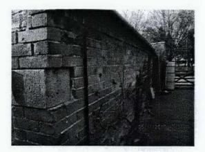
The elevation has suffered outward movement arising from roof-spread. Whilst plumb and vertical to within normal construction tolerances at the corners of the building, reconstruction of the remainder of the elevation is advisable, unless it can be buttressed satisfactorily by the proposed link between the buildings.
