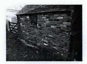
5.2.3 The rear gable wall is plumb and vertical with no indications of structural movement.
