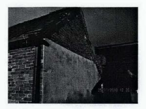
3.2.4 The roof of the end-bay is of single timber purlin construction, the rear purlins approximately 200mm x 150mm and the front approximately 175mm square with chamfered edges. The rafters are typically 150mm laid flat with sawn timber battens supporting plain clay tiles. The rafter feet bear on large 100mm deep timber wall plates.
