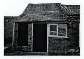
The gable wall has exposed original 110mm half brickwork to the apex. This shows a slight outward lean, although not sufficient to threaten structural stability. The brickwork is in need of repointing and the cutting out and replacement of weathered bricks. The main lower section of the wall has a modern render finish which is undecorated. It is in sound condition, although in contact with underlying concrete and damp affected at the base.
