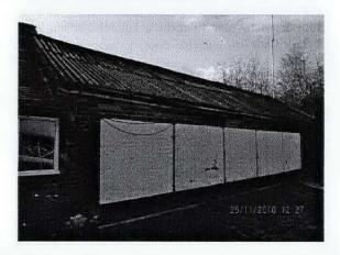
Mortar pointing is generally satisfactory, although making good defective mortar and weathered brickwork to the left hand gable wall will be required in conjunction with refurbishment works.
