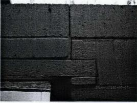
The front and gable walls are plumb and vertical to within normal construction tolerances.
