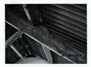
The present lightweight roof covering is adequately supported despite these defects. Nevertheless, it is anticipated that provision of a traditional tiled roof covering will demand replacement of the purlins and the raising of the truss bases to create improved headroom.
