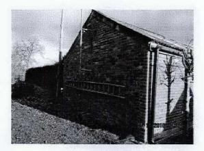
The line of the rear wall does show a curve and an inward lean at the eaves to the centre of the elevation. This coincides with truss bearings suggesting that the damage was caused by the cranking of the original roof towards the front of the building. This will have resulted in the probable outward curve of the front elevation, the principal reason for its reconstruction. Completion of the latter has stabilised the rear wall.
