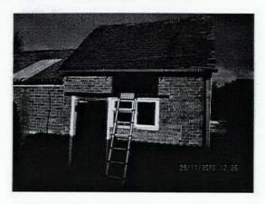
Internally the bay is sub divided by internal 225mm brick wall and by short 110mm half brick wall extending from front to rear to form a kennel kitchen and two storage rooms. The building has a loft floor with low external doorway opening.
