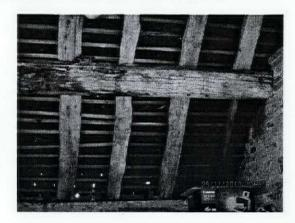
The purlins and rafters are affected by active beetle infestation and the exposed purlin ends by wet rot. Conversion and refurbishment of the building may be expected to demand replacement of the roof timbers. Nail fixings of timber battens have corroded giving rise to evidence of slippage, particularly to the verges and eaves, and at the rear. A cement fillet provided at the junction of the main building has deteriorated, giving rise to consequent penetrating dampness in the rear storage room.
