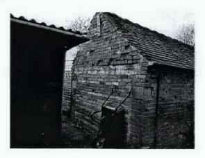
The gable apex has suffered outward movement and a steel pattress plate restraint has been applied with rudimentary wire fixing to a short timber spanning between facing rafters.
