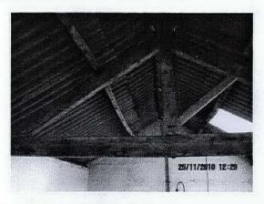
The trusses are structurally sound, albeit with localised active infestation by common furniture beetle, although a single strut has been lost with reinstatement required.
