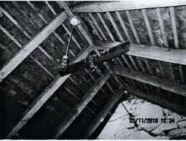
The infill brickwork to the underside of the timber beam is in sound condition.
